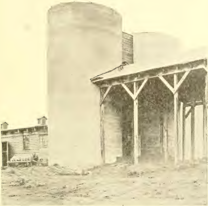
Two of the Four Silos on the Dairy Farm of Thomas A. Edison, at Stewartsville, N. J.
